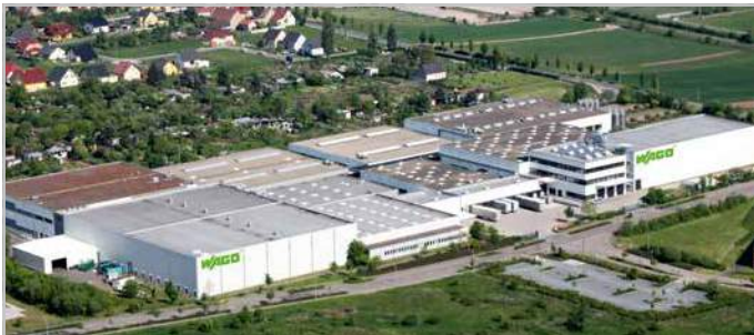
WAGO Sondershausen, Germany
