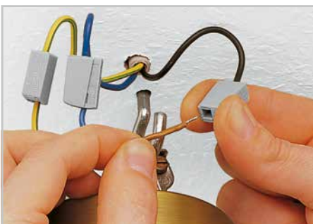
Lighting side: Press button fully, insert stripped conductor into square entry and release.
